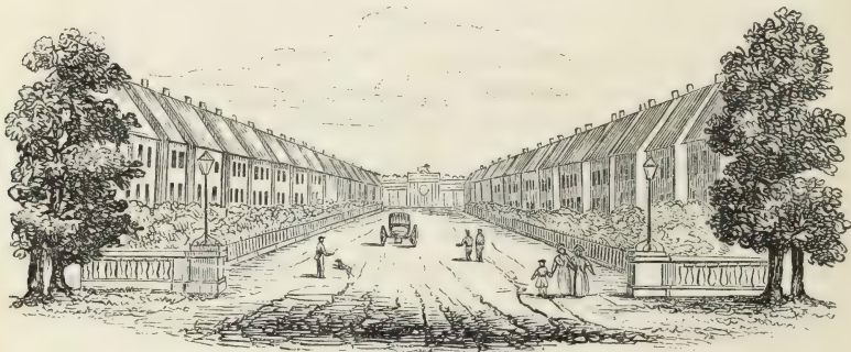
[Fig. 86. View of the town of Harewood, shewing the gateway to Harewood Hall at the farther end.]
